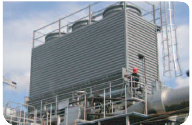
:: Central Sugar Refinery Selangor, FRP Pultruded Structure, 600 HRT.
